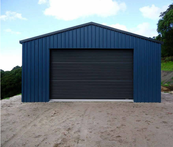
ROLLER DOORS TO BOATSHED
