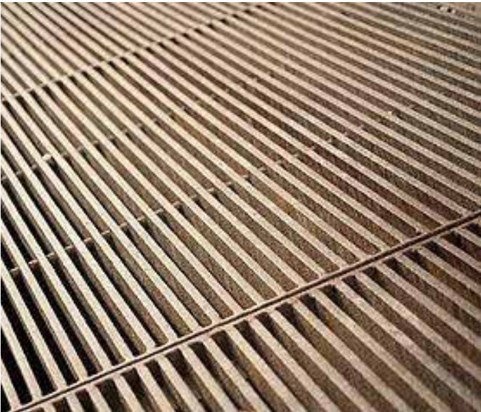
FL MS UPPER DECK FLOOR FINISH: STEEL GRATE
